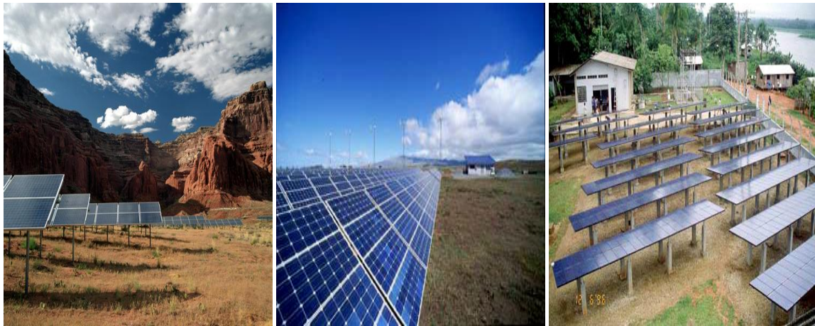
Figure 1.9 Peneaux solaire installé à: a) Rope Marina b) Parker Ranch c) Brazil
