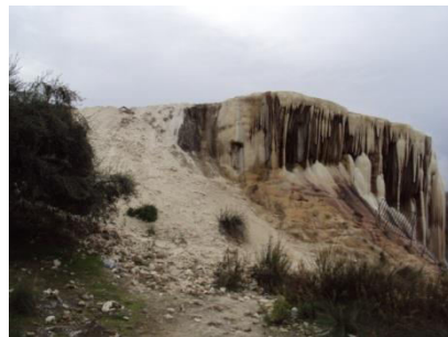
Fig .9: The collapsed
